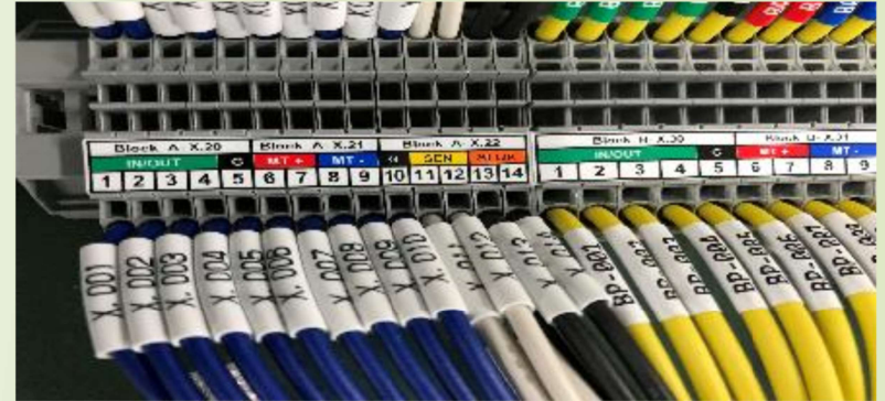
`Push-in` Type Terminal Block
